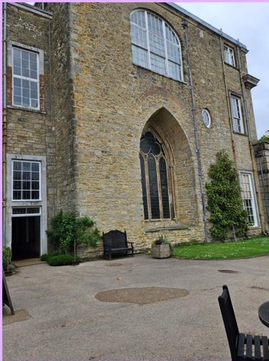
The Chapel – the Oldest Part of the House
